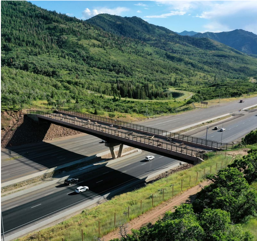
Transportation Solutions Wildlife Crossing Bridge project
