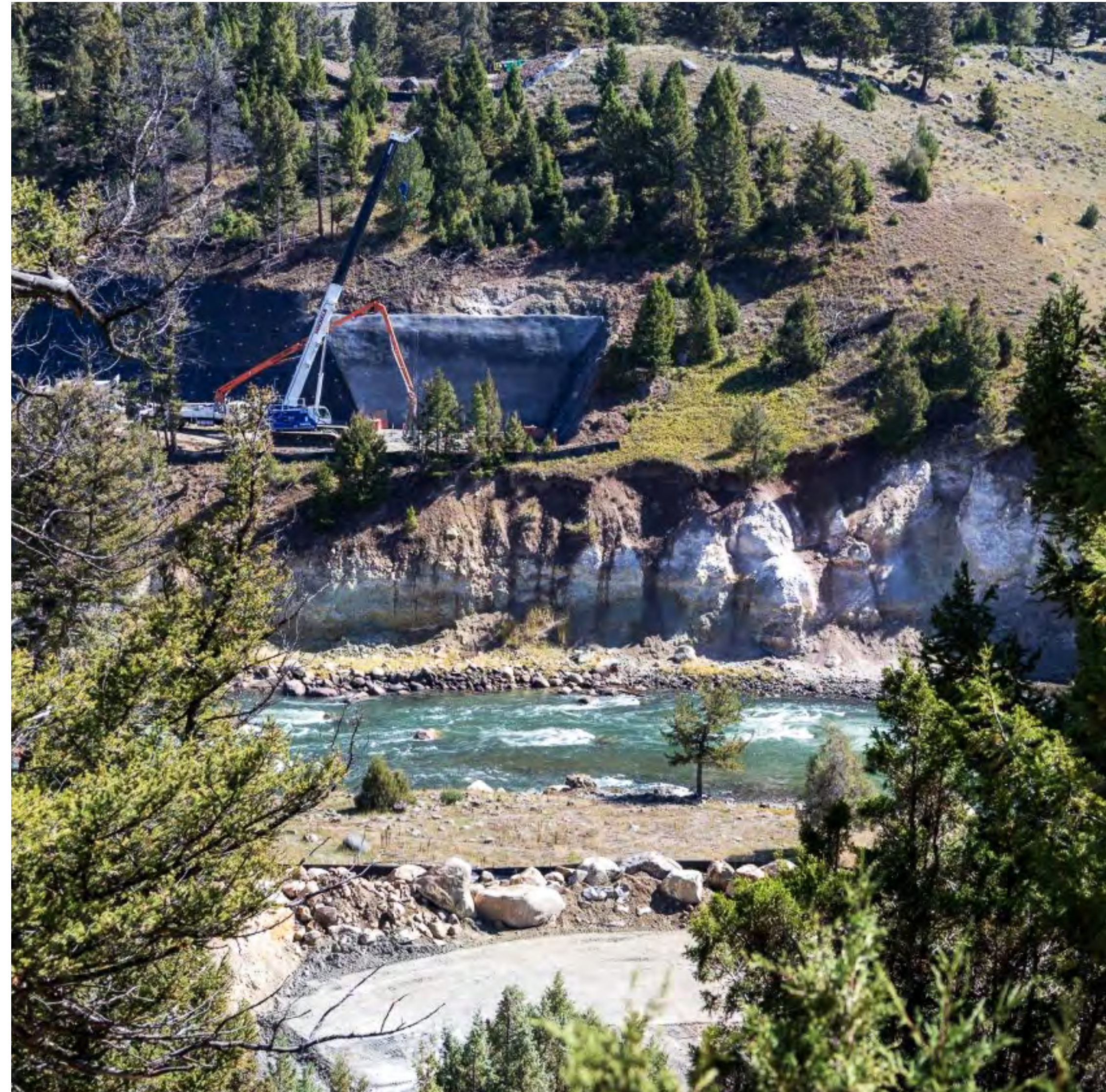
RLW (Transportation Solutions) project site
