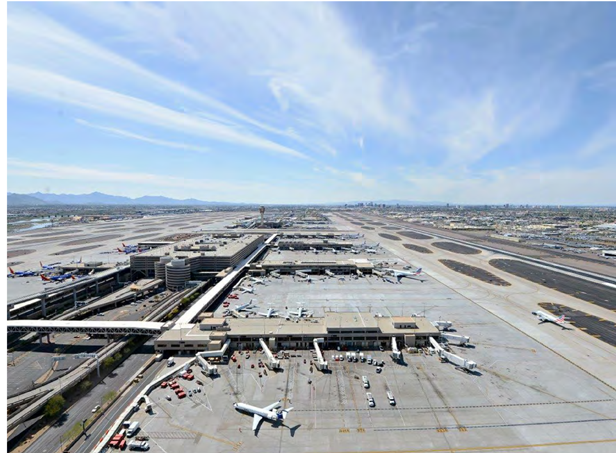
Banicki (Transportation Solutions) project site
