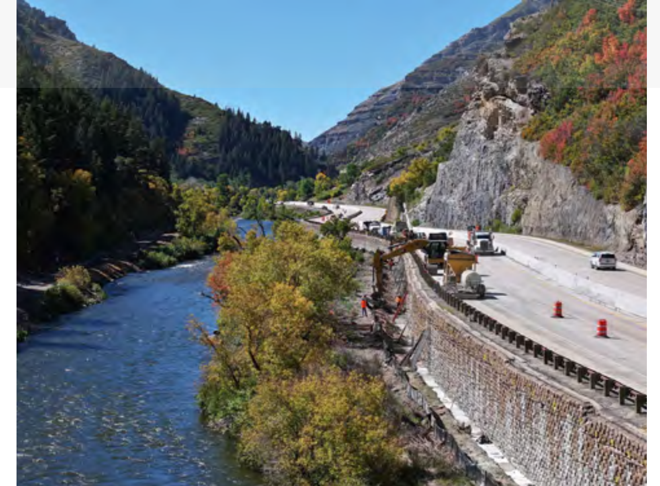
RLW project along the Provo Canyon
